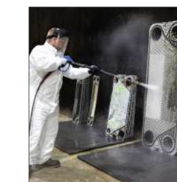
HEAT EXCHANGER CLEANING, REPLACEMENT, & SERVICING
